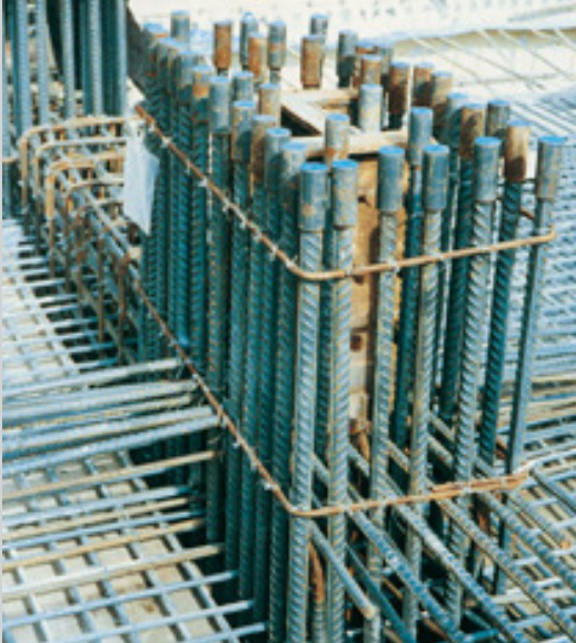
Column Construction using Tapered Thread Couplers
